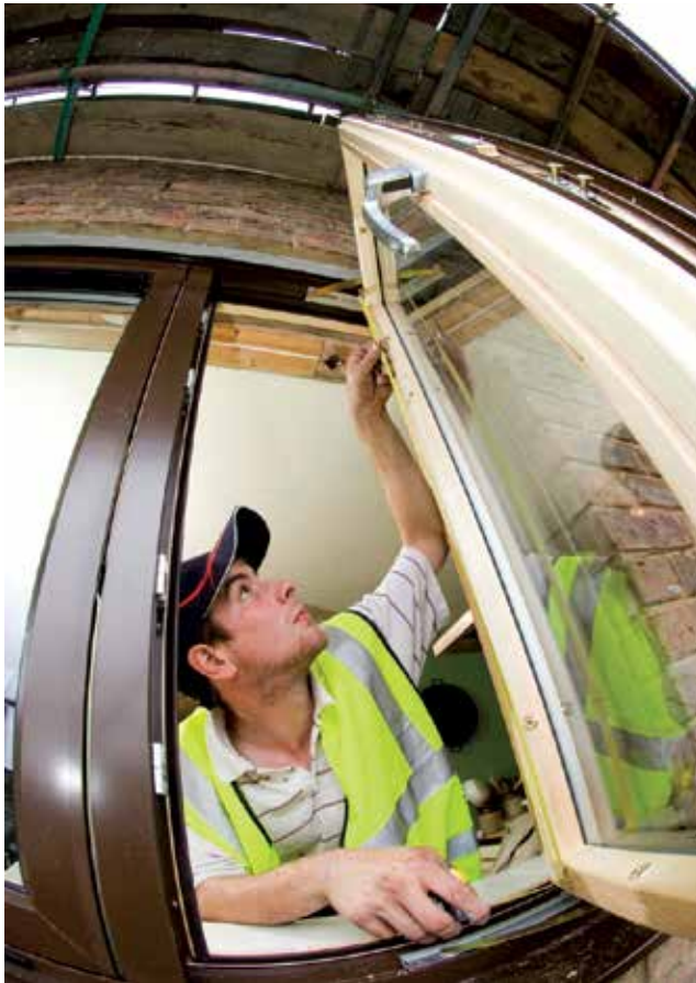
Repairs getting underway
